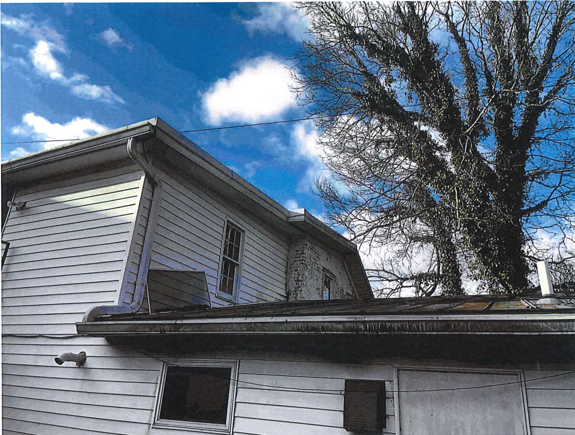
The rear exterior wall of the original building has no damage.
