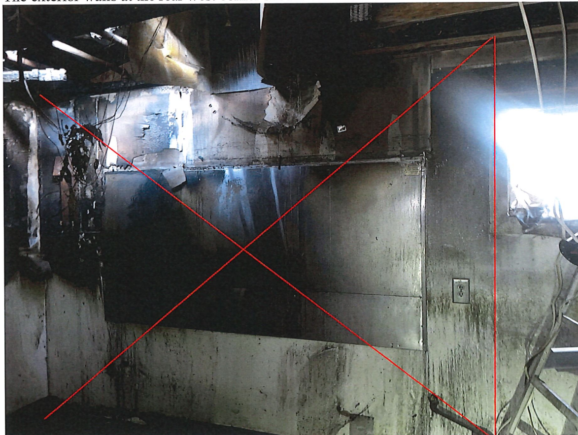
The exterior walls should be rebuilt between the windows.
